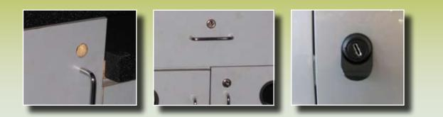
Above pictures illustrate a typical disc tumbler cam lock installation after only one year in a high-use environment.
